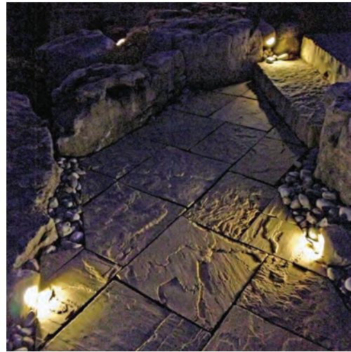
◀ These custom-made lights were created out of cored-out limestone so the lights could be hidden while safely lighting the potentially dangerous stairs. PHOTO BY SEAN JAMES.
